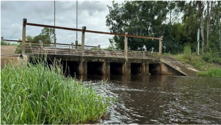
图2 A1管理区水闸 Fig. 2 Sluice gate in Management Zone A1
