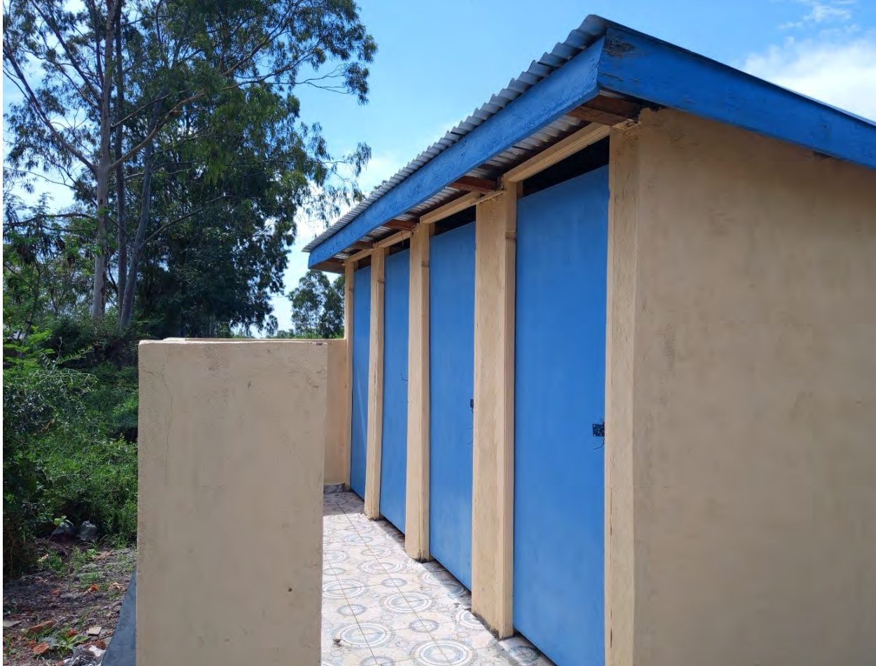
Image 7: Pit latrine was constructed at a school in Kisumu.
