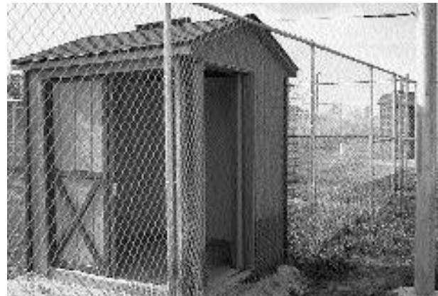
Fig. 12.10. Chain link fence. Photo also illustrates 0.5 m tall chick guard, and Patuxent's new double-door, feed/wind shed.
