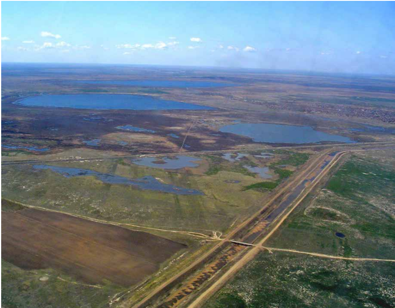
Canals and roads constructed within Zhalong National Nature Reserve alter water flows in the core area, reducing and fragmenting breeding habitat (Photographer: Liying Su)
