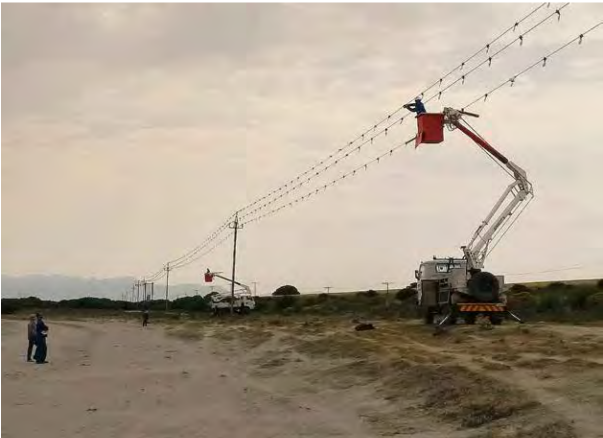
Marking power lines in South Africa to reduce collisions by cranes and other birds (Photographer: Constant Hoogstad, Endangered Wildlife Trust)
