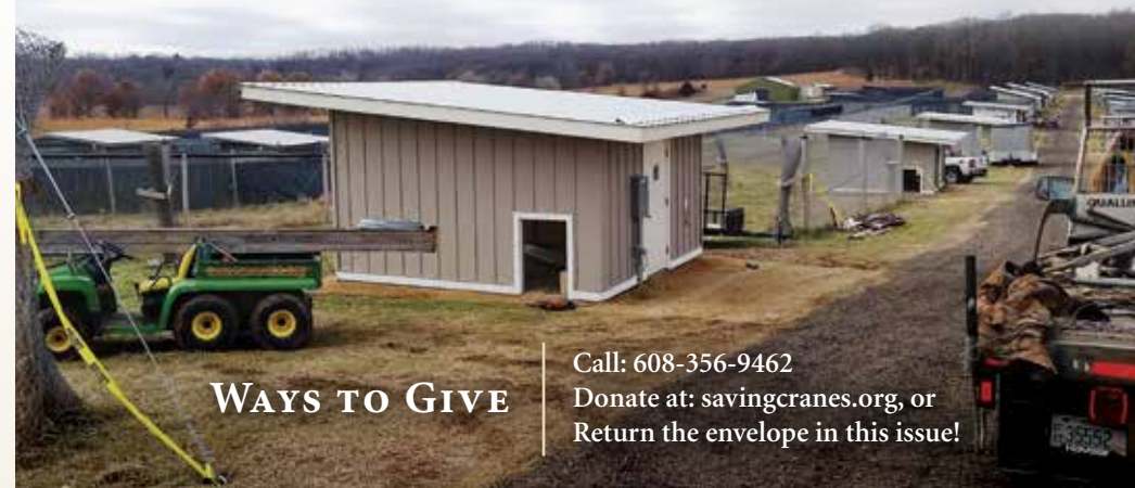
New and remodeled cranedominiums line the streets of Crane City. Your donation will help us continue this work.
