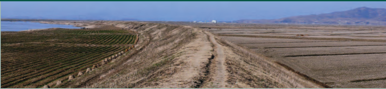
High dikes prevent the Namdae River from inundating the rice fields that once provided waste grain for wintering Red-crowned Cranes.
