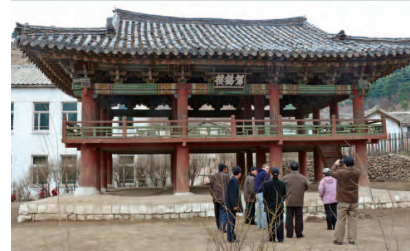
The Ga Hak Lu (Crane Watching Pavilion) was built between 1735-1742 and was a part of the Anbyon Guest House where travelers could find lodging. The architecture is simple and the building is one of the oldest in Democratic People's Republic of Korea (DPRK). Can you imagine sitting on the elevated platform and watching Red-crowned Cranes on nearby wetlands while warmed by spicy kimchee and thick blankets?
