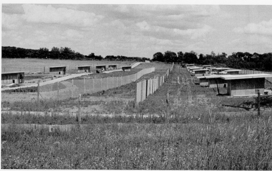
As the initial phase of "Crane City" nears completion, ICF's 24 new "cranedominiums" are readied. A service building will follow. Photo by Marion Hill.
