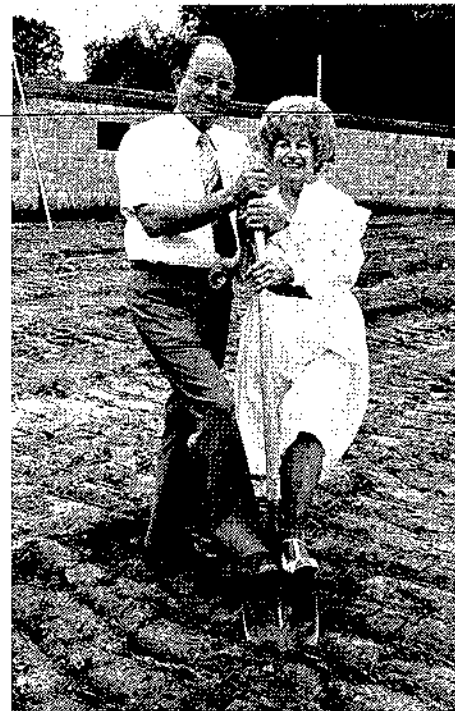
Norm and Claire Sauey begin the excavations for the Sauey Hatchery, named in their honor. photo by Jeff Strobel-Baraboo News-Republic
