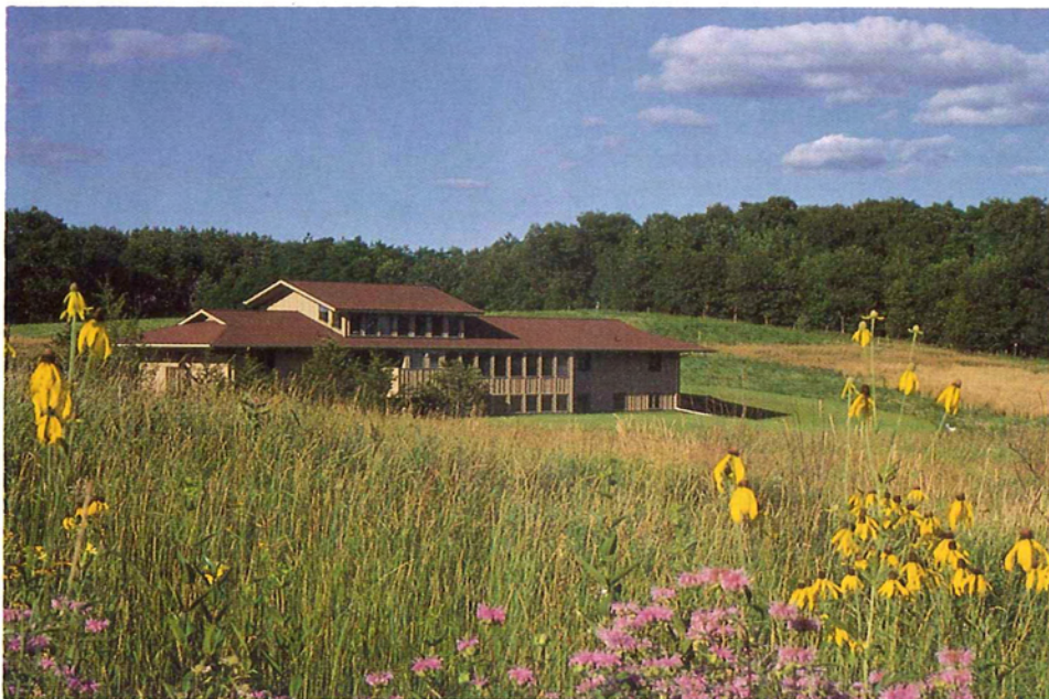
ICF's new Scott International Guest House and Stedman Training Center sits beside ICF's prairie restoration. As home for ICF interns and foreign colleagues, the Guest House provides a place for different cultures to get acquainted. Photo by David Thompson.
